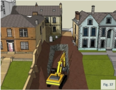
1) Ground between Talbot and York House excavated, leaving banks of ground to provide continued support to foundations
